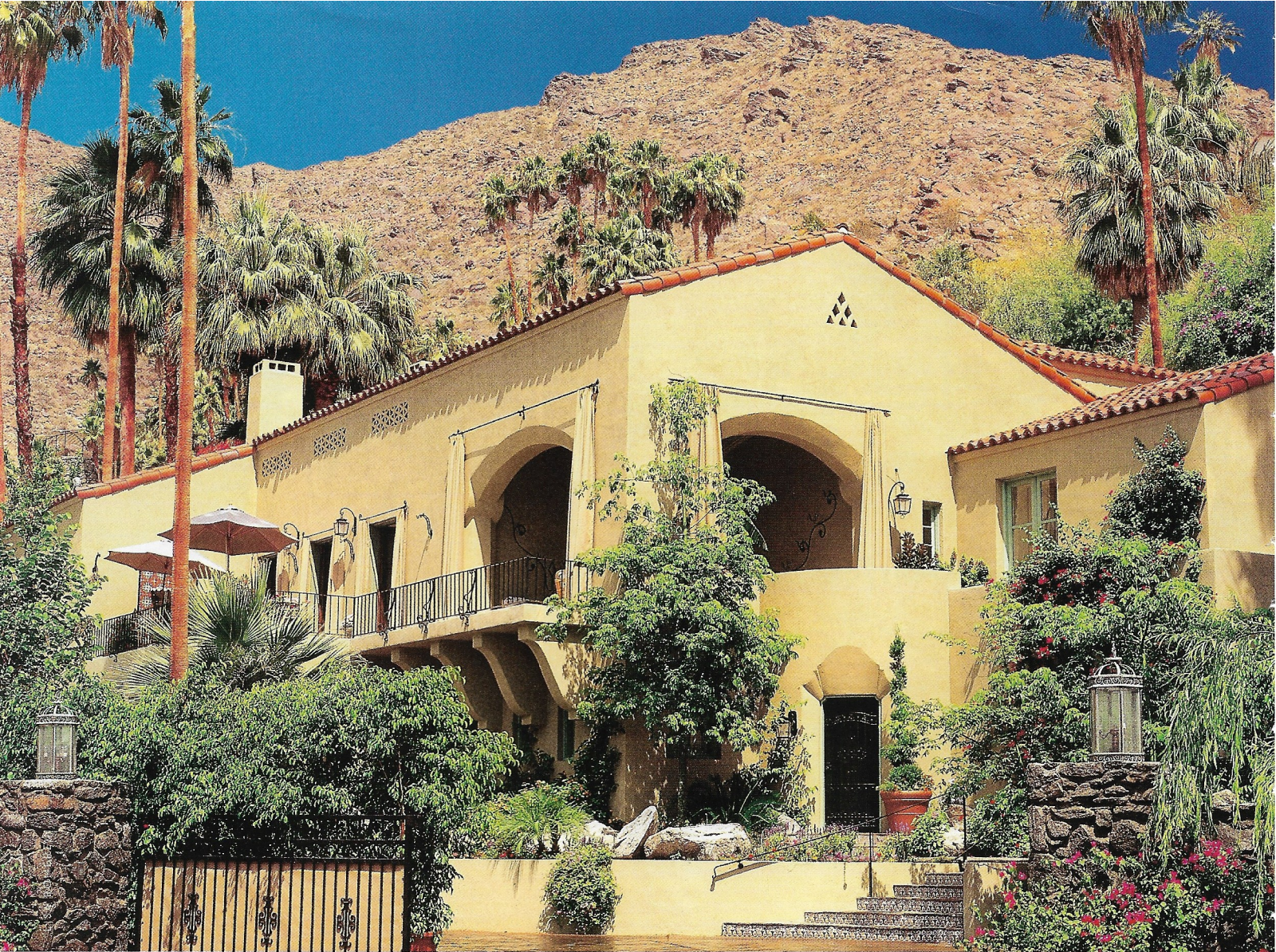
The Willows today. A private residence when it began life in 1925, it was saved 70 years later by Tracy Conrad and her husband, Paul Marut.
